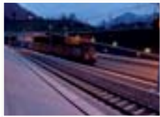
BLS Cargo drives the first trains through the new Lötschberg base tunnel in 2007.
